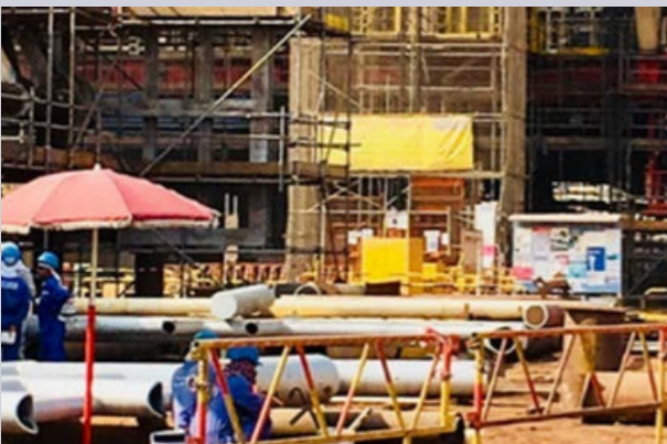
Future Pipe Factory
